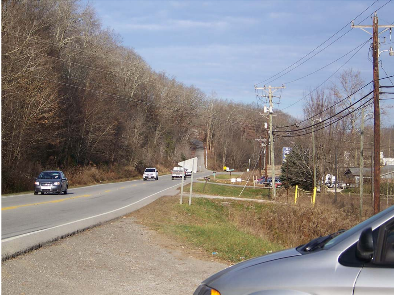
KY 32 going West past Copperas Hollow Rd. Limestone Rd. seen ahead intersects at an skewed angle and causes sight distance problems.
